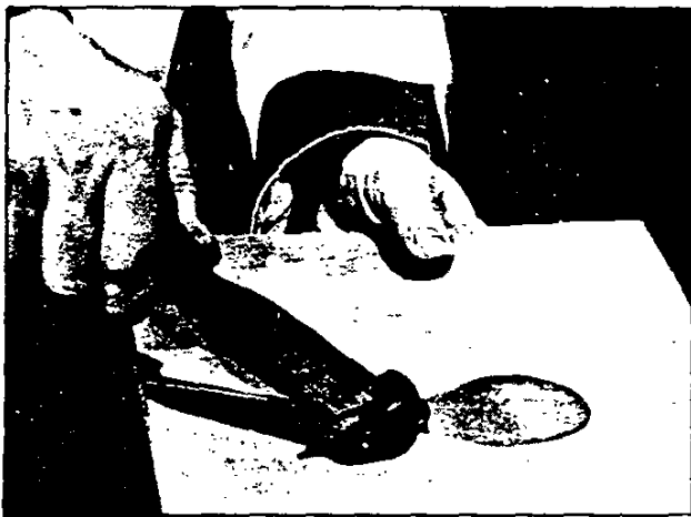
Fig. 54—Mixing Plastic (Epoxy) Solder Material
